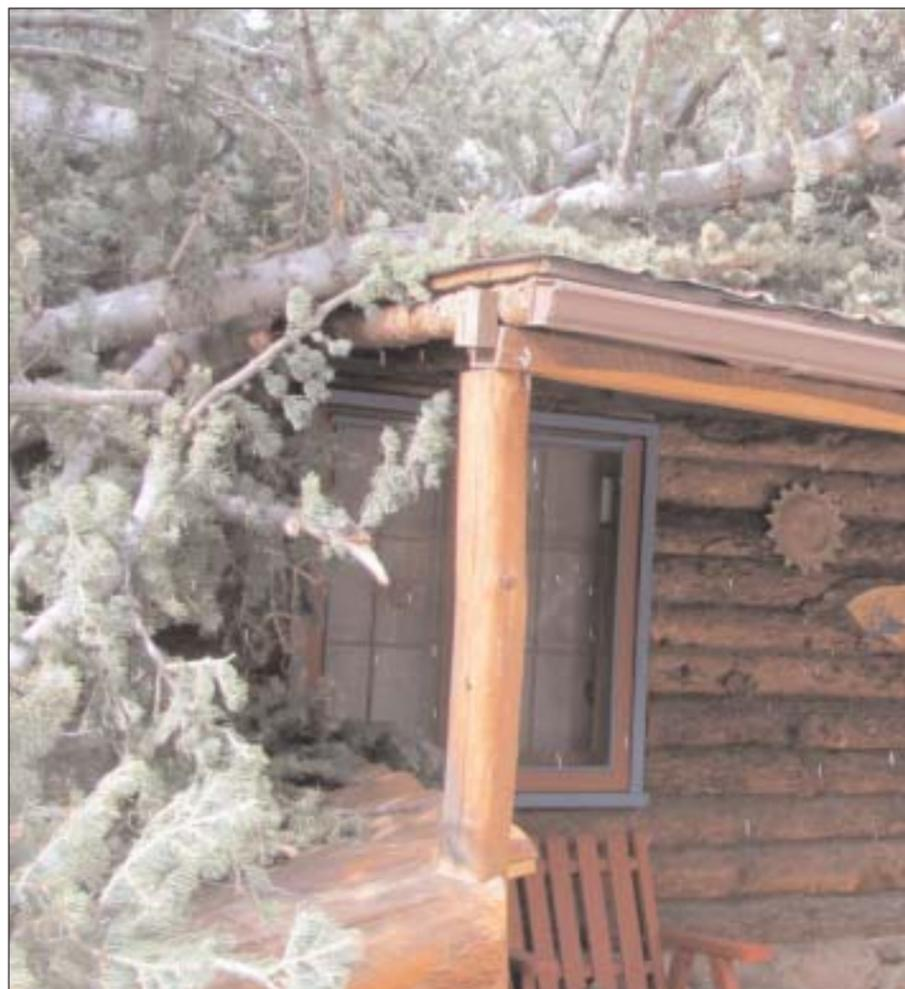
Two fir trees snapped off about 12 feet up and landed on the roof and porch area of this cabin - luckily the cabin walls did not collapse and fortunately the branches broke off and did not pierce the roof. *Photo by JVA*
